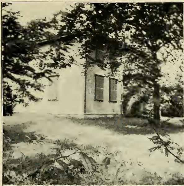
Bedford Street, near the Green
